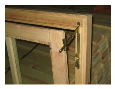
The window will then tilt slightly inwards at the top for ventilation.
